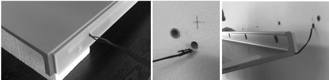
12. Connect the power cord to the controller. You then connect the controller to the driver. Plug the plug attached to the driver into the wall socket.
